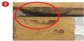
1 Wanes (chippings) are not allowed on the stringer boards (middle, side).
