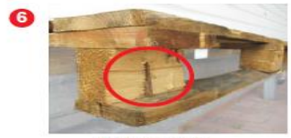
6 Chipped block, exposing any nails.
